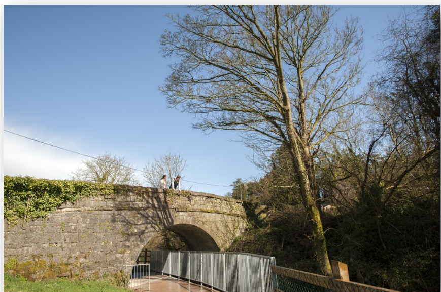
Ulster Canal, Phase 1
