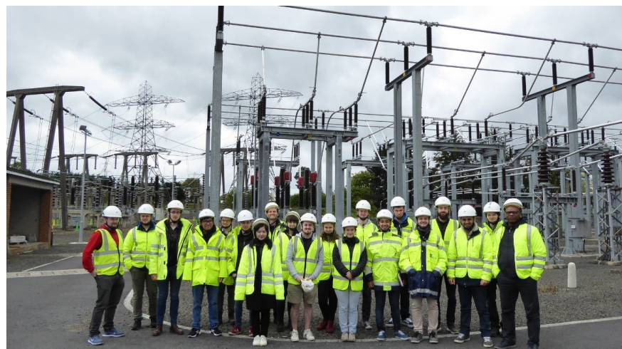
Visit by Queens University Belfast SPIRE 2 team and associates to NIE Networks' Castlereagh Substation (275 KV) on May 3rd 2019.
