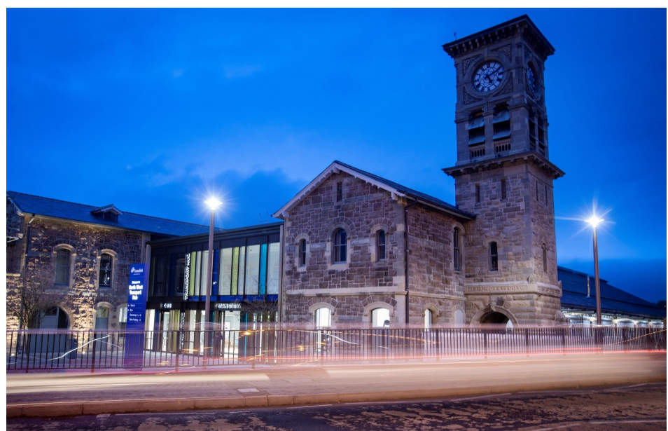
Exterior of the North-West Transport Hub
