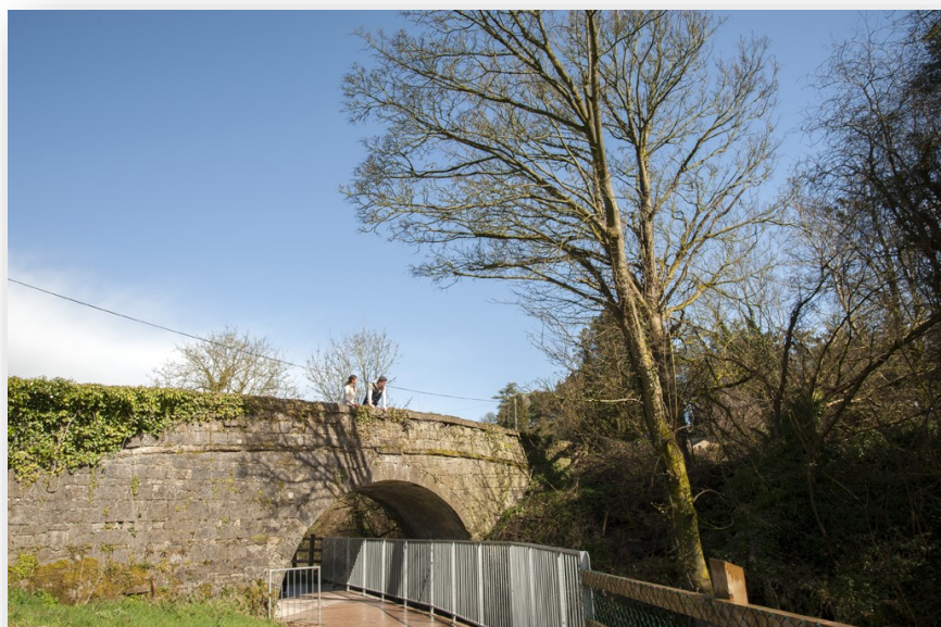
Ulster Canal, Phase 1
