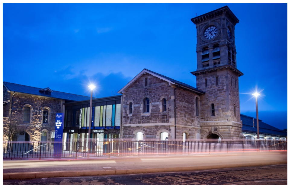
Exterior of the North-West Transport Hub
