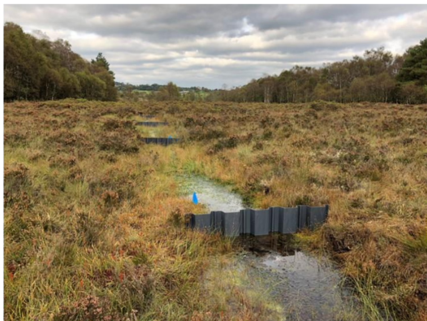
Figure 3.1: Fairy Water Bog drainage blocking
