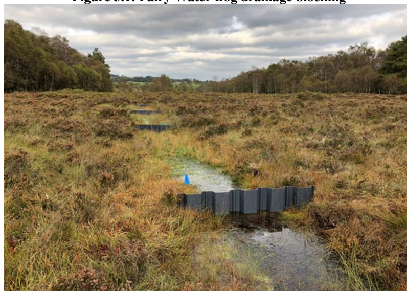
Figure 3.1: Fairy Water Bog drainage blocking
